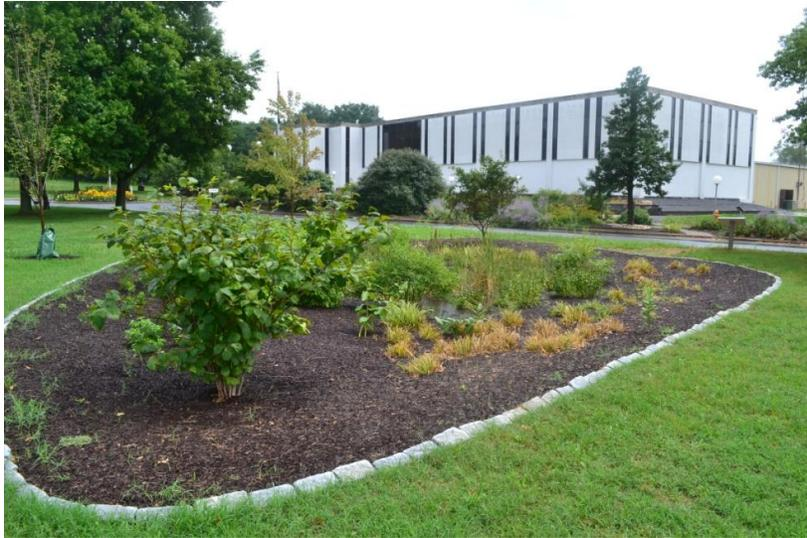
A rain garden, like the one at the Berks County Agricultural Center, catches rain water runoff and allows it to be absorbed into the ground where it can be used by native plants. It also helps to infiltrate stormwater back into the ground. This helps to recharge groundwater levels and to reduce the amount of pollutants from reaching lakes, streams and rivers.
